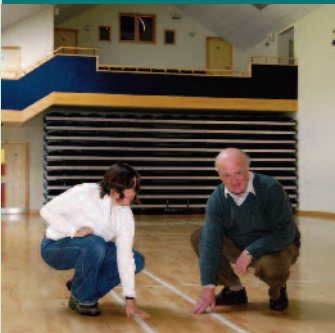
Underfloor heating in main hall
