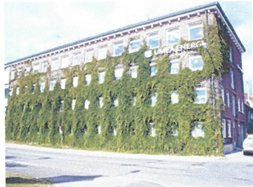
The headquarters of Umeå Energy, which provides heat and electricity from residential solid waste.
