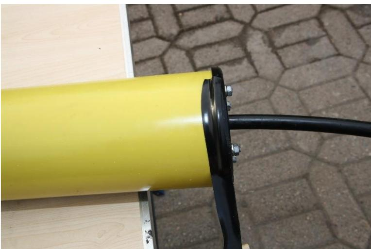
Install two rounds of vulcanized tape on each end.
