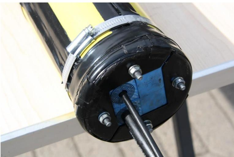
Finally, tighten the nuts of the pass-through frames at the ends of the joint closure. Tightening should be done carefully to ensure that the pass-throughs are properly sealed.
