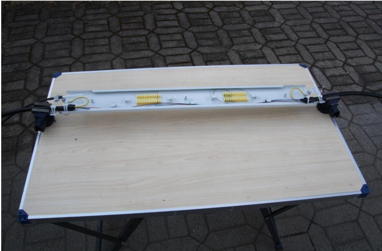
The cables have been attached to the splice tray and the branched fibers have been spliced. Finally, to protect the fibers, secure the plexiglass cover that comes with the splice tray.
