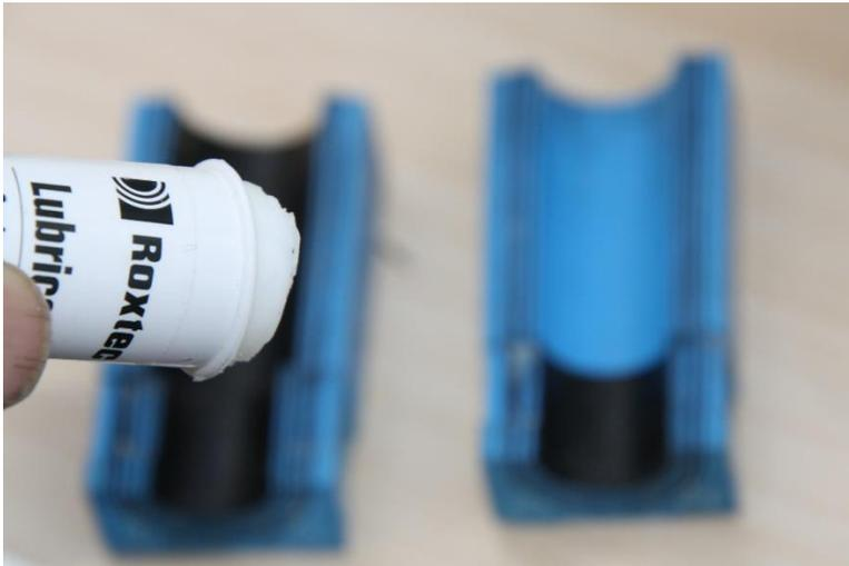
Carefully lubricate the outer and inner surfaces of the RM modules with the lubricant that comes with the package.
