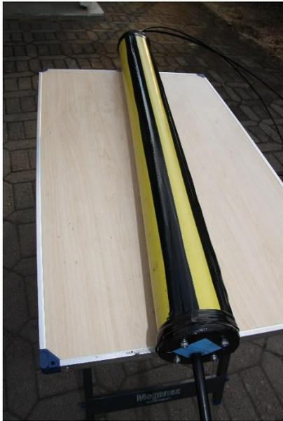
Tape the seams of cable tubes and finally another round to the ends of the extension.
