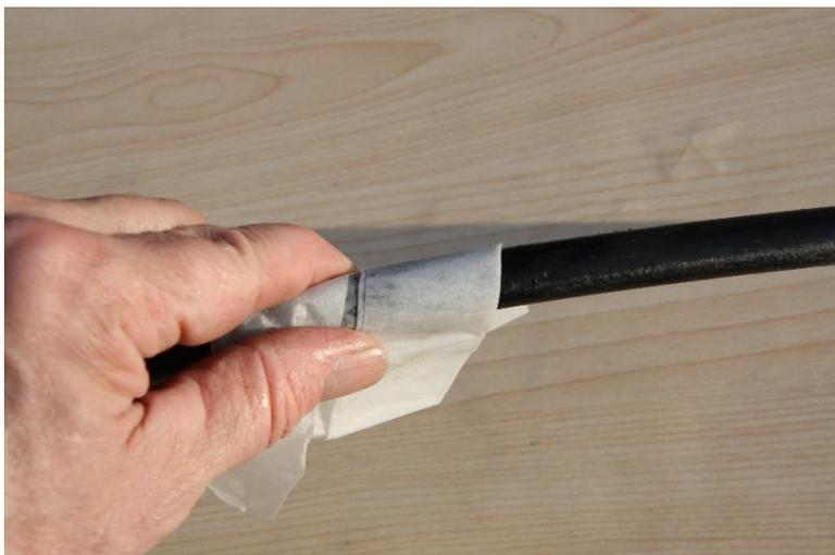
Clean the surfaces of the cables carefully, outwards from the ends of the cable sheaths. For cleaning, you can use the cleaning wipe that comes with the package.
