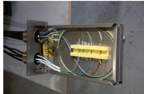
The fibers are measured on the upper splice tray before splicing.
