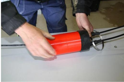
Pull the frame tube on the splice tray along with the rubber cable glands.
