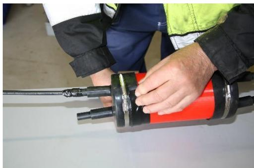
When the beginning of the tape sticks, turn the tape around the case while slightly stretching and pressing it into place.
