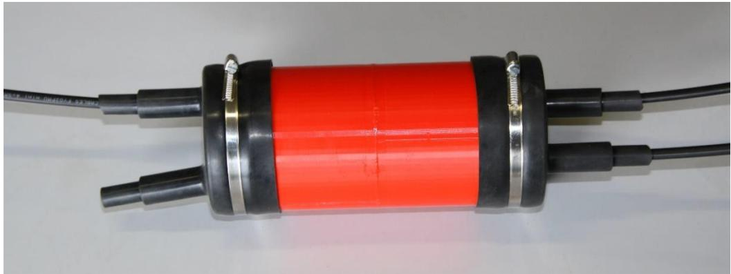
Lock the end pieces to the frame tube with the hose clamps that come with the joint closure. When installing the hose clamps, note that they are straight and between the raised stripes at the ends of the frame tube!
