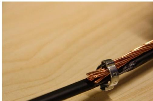
Position the hose clamp in a way that makes sure sufficient connection is made. Flatten the end of the grounding wire and place it between the cable and the hose clamp.
