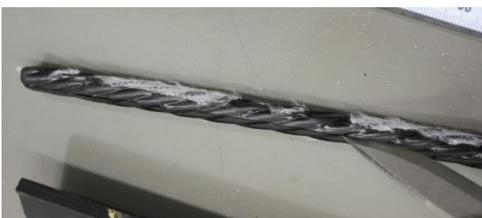
Carefully make a longitudinal incision to the middle sheath between 10 cm and 15 cm in length. Do not cut too deep to prevent damage to fiber tubes.
