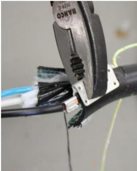
Flatten the end of the cable sheath with pliers and squeeze the connector of the grounding wire onto that half of the sheath.
