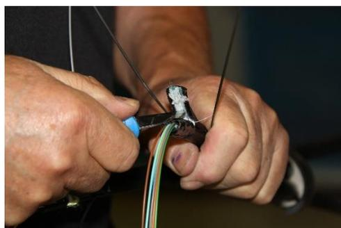
Use a knife to scrape off the white ribbon under the armoring from one of the halves of the cable sheath. Also scrape off the plastic layer on the surface of the armoring.
