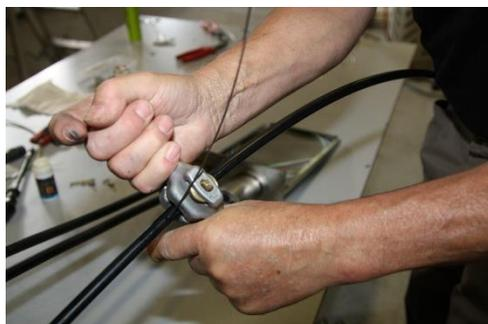
Split cable sheath using ST-OCS splitting tool. Guide the tool blade into the groove of the steel wire and pull the sheath open on both sides of the cable.
