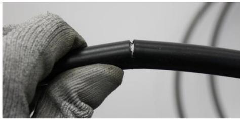
Bend the cable in different directions at the incision point to break the steel band.
