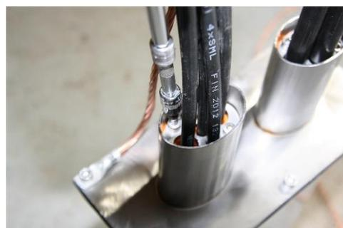
Check the tightness of the screws in the cable glands using hand tools.
