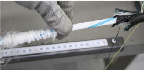
Pull the binding threads as bundle off the fiber tubes.
