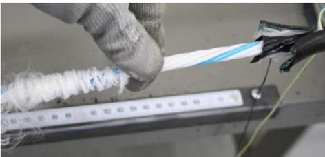
Pull the binding threads as bundle off the fiber tubes.
