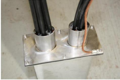
If cables containing metal are brought into the closure, the closure must always be grounded.
