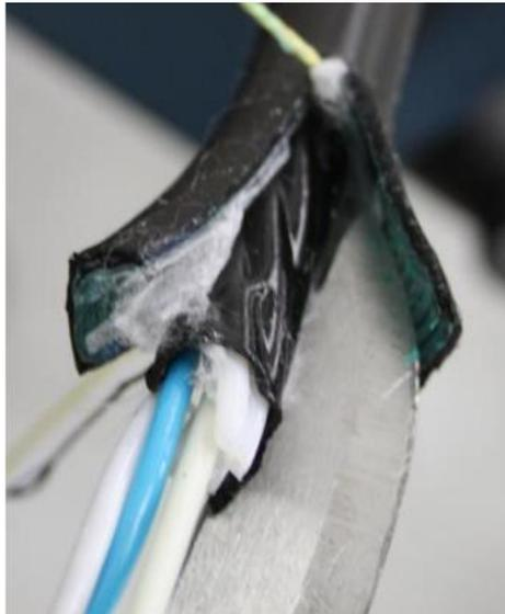
Scrape off the white ribbon under the armoring from one of the sheath halves and the plastic layer on the surface of the armoring.
