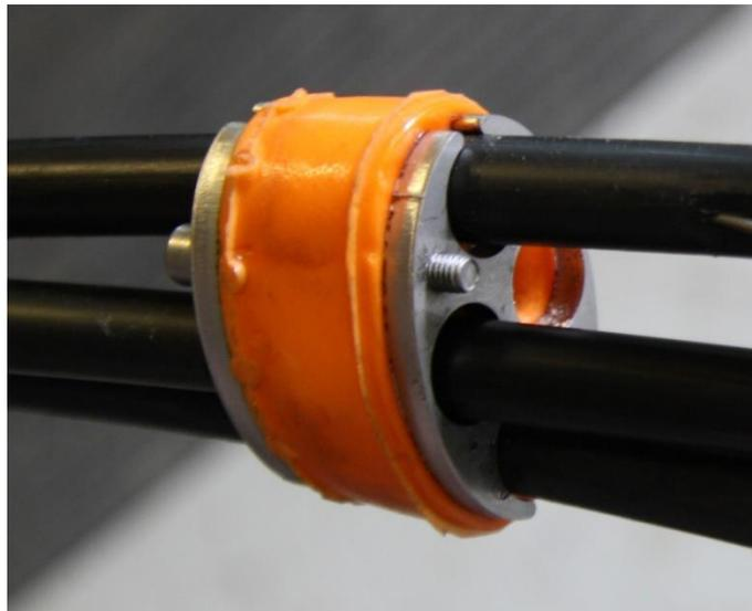
Cables brought through a 4-hole cable gland
