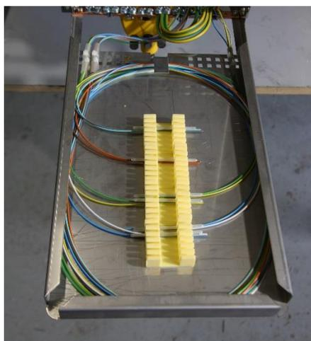
The fibers are measured on the splice tray before splicing.
