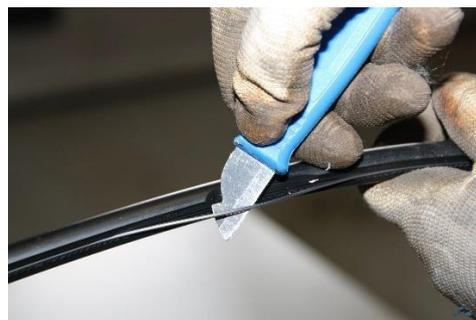
Dig out the steel wires.
