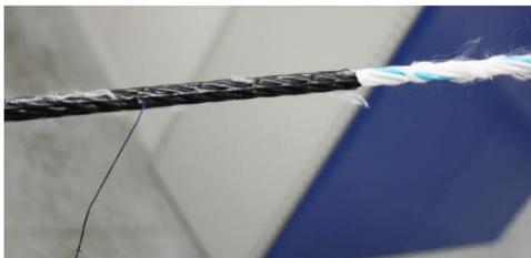
Cut off the bended section without damaging the tear wire and split the rest of the sheath using the tear wire
