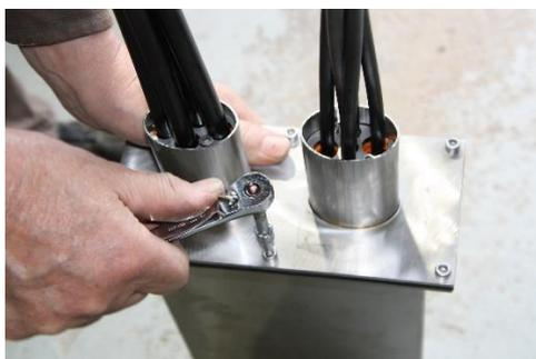
If you are using a battery-powered screwdriver to tighten the screws, finally use a hand tool to make sure that the joint closure is securely closed.
