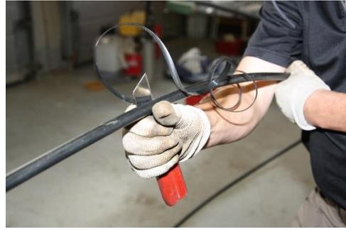
Peel the sheath off the steel wires, either for about 50 cm or for the entire length to be peeled.
