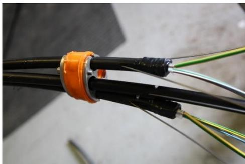
FZVD2PMU Flex direct buried cables in a mechanical cable gland.
