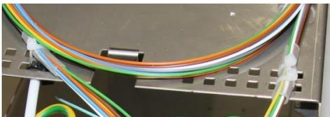
Attach the uncut fiber tubes to the splice tray with split silicone tubes and cable ties.
