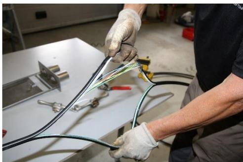
Pull the cable halves apart while taking care not to damage the Flex fiber tubes. If you have opened the cable for only a short distance, carefully pull the Flex-tubes out as a bundle from the outer end of the cable
