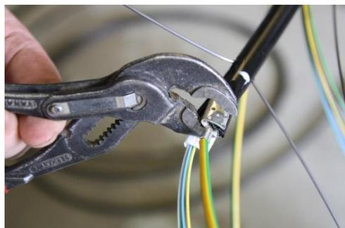
Flatten the end of the cable sheath with pliers and squeeze the connector of the grounding wire onto that half of the sheath.
