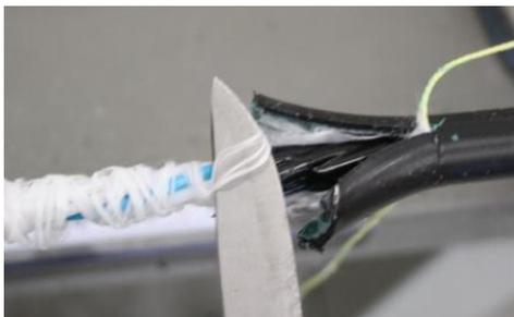
Push the binding threads of the fiber tubes towards the cable to loosen them, and cut them at the base of the sheath.
