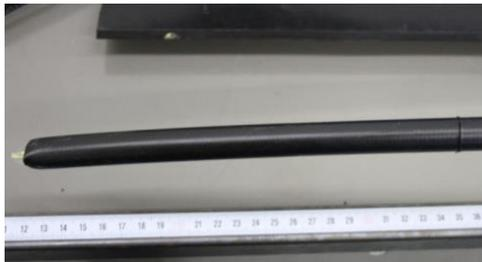
Use the knife to cut around the cable sheath up to the steel band at a distance of approximately 15 cm from the end of the cable.
