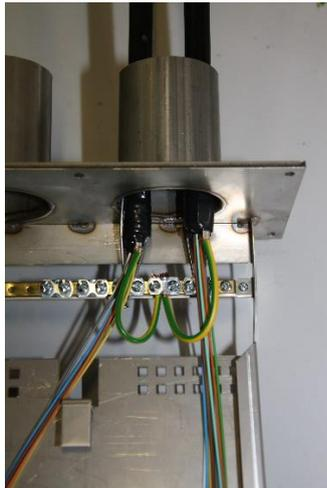
Connect the steel strength members and grounding wires of the cables to the grounding rail of the closure.
