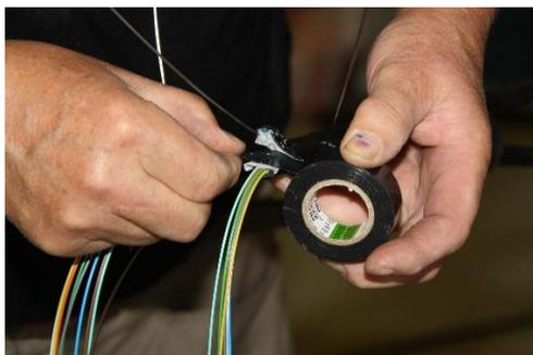
Bend one of the halves of cable sheath and press the Flex-tubes inside the white ribbon against it. Protect the tubes by wrapping insulation tape around the tubes and the cable sheath half.
