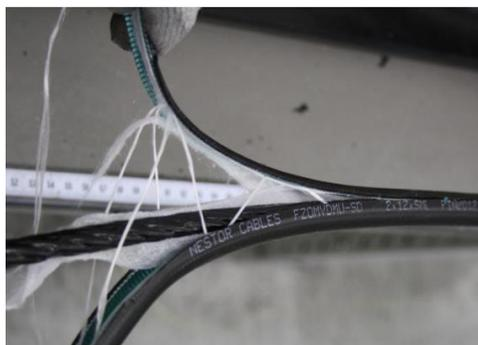
Pull the sheath open to the starting point of the peeling.
