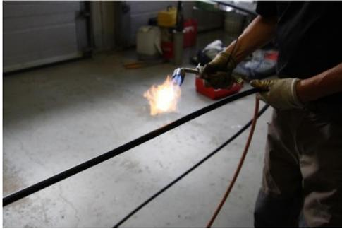
Clean the cable from any dirt and heat the cable sheath over the entire length to be peeled. This makes peeling easier, as the cable sheath material is HDPE, which is harder material than the LDPE traditionally used in outdoor cables.
