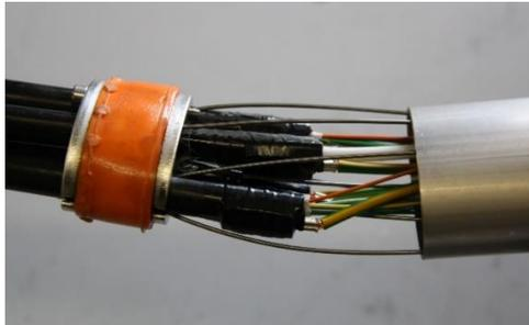
Guide the cables with fibers, steel wires and grounding wires as a bundle inside the joint closure.
