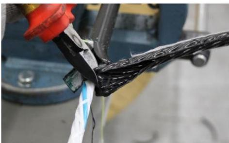
Pull the split sheath off the fiber tubes and cut it under the halves of the outer jacket.
