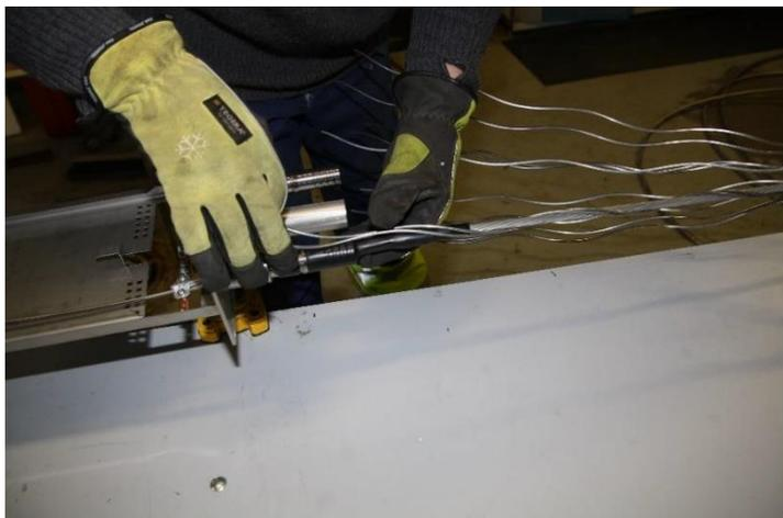
Place OPGW's outer wires individually and in its own order on top of the cable pass-through.
