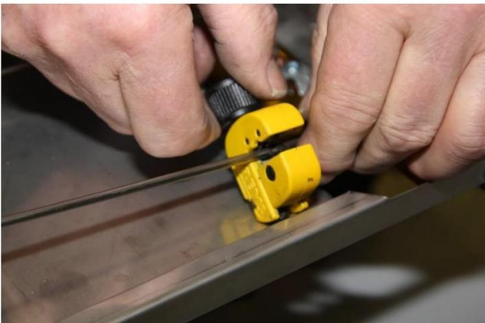
Carefully cut the steel fiber tubes with a pipe cutting tool.
