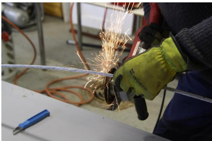
Make grooves on the outer wires of the OPGW either with an angle grinder or a hacksaw.
