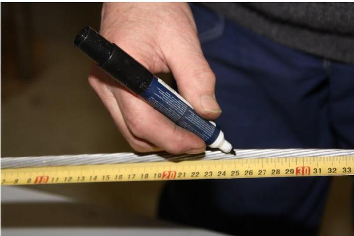
Mark the sealing point on the yarns of the inner layer at 25 cm backwards from the cutting point of the wires.
