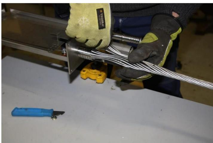
Try to get the wires as evenly as possible over the cable pass-through.
