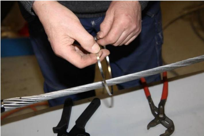
Lock the wires to the pass-through with the steel cable ties that come with the joint closure. Both OPGWs must be locked with at least three steel cable ties.
