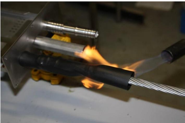
Pull the top shrink all the way to the joint closure and shrink it into place.
